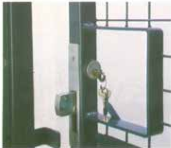
Standard Dead Bolt lock installed in a typical sliding gate showing positive gate stop. Lock cylinder accessible from both sides of gate.
