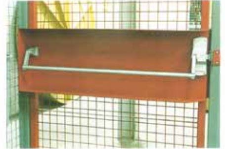
Standard panic bar attachment installed in typical swing gate.
